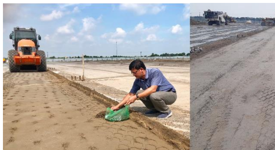
Figure 7. Application of dredged material for building foundation of cargo yard in Hai Phong, Vietnam
